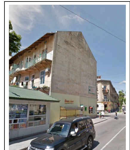
Fig.2. Blank façade in Lviv [Google Earth]
