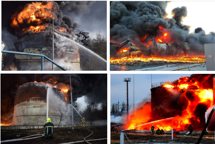
Fig. 2.3. Fire situation at the oil depot as a result of shelling
