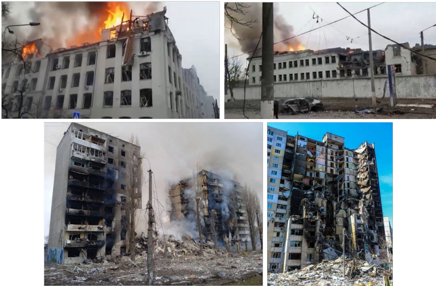
Fig. 2.9. Damage to civil infrastructure objects as a result of shelling, which are accompanied by fires and destruction
