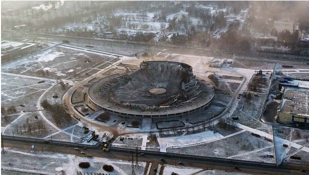
○ Fig. 1.10 Collapse of the St. Petersburg sports complex, January 31, 2020
