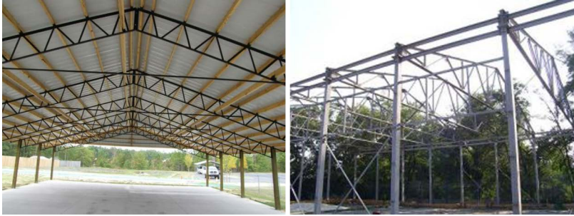
○ Fig. 1.3 General view of the steel truss
