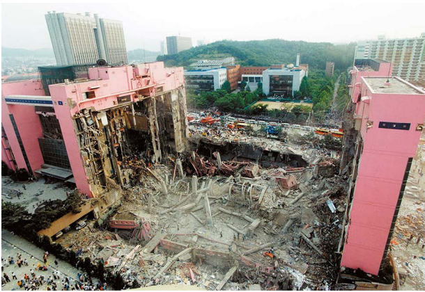
○ Fig. 1.9 Collapse of a 5-storey supermarket in Seoul, 1995
