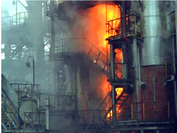
Fig. 1.5 Fire at the Saratov Oil Refinery on October 4, 2012
