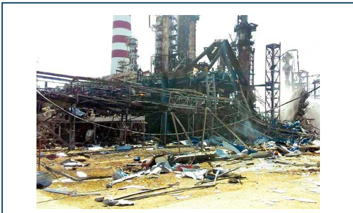
○ Fig. 1.7 Destruction of structures because of the accident at the Achinsk refinery in June 2014
