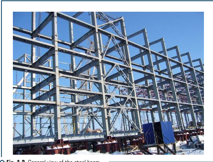
◉ Fig. 1.2 General view of the steel beam
