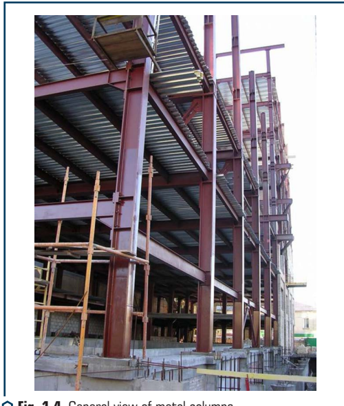
○ Fig. 1.4 General view of metal columns
