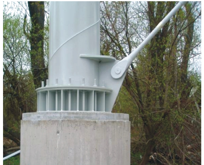
Fig. 5. Anchoring of the pylon – proposal and realization
