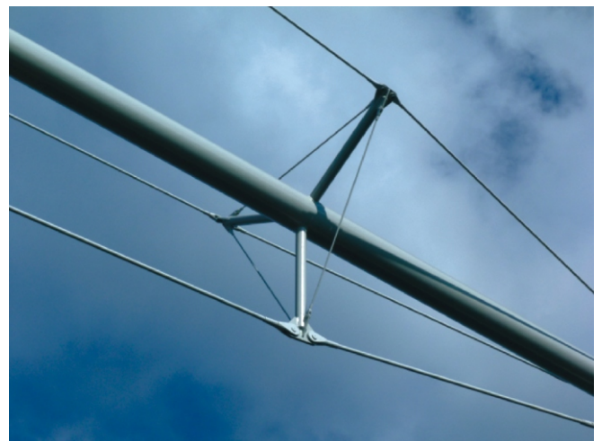
Fig. 7. Cross-frame beam – spatial beam string structure
