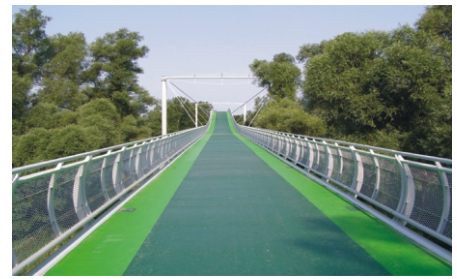
Fig. 14. View on finished bridge
